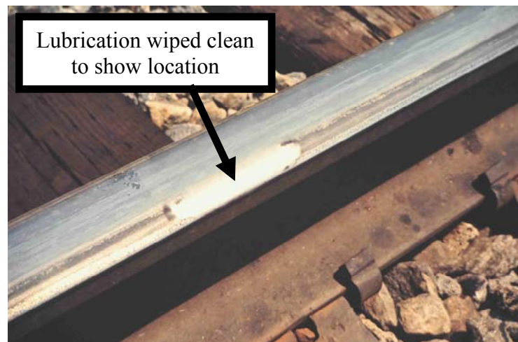
Figure 29, Typical rail lubrication in the field
